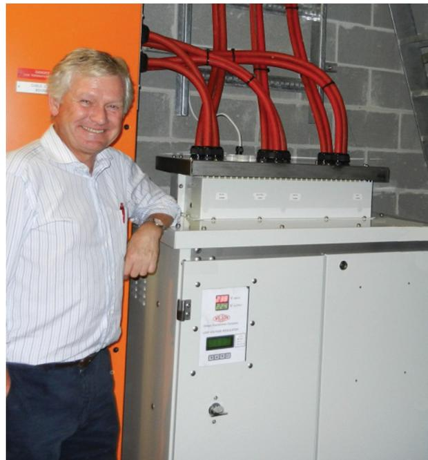
Wilson's 750 kVA Voltage Power Optimiser installed in Melbourne
