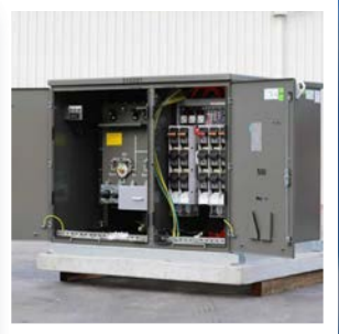
Compact MV Substations
